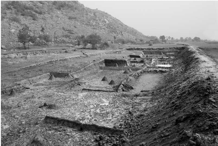
A percolation tank for holding local runoff under construction in Koilu watershed
