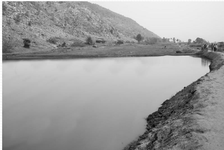
The above percolation tank filled by local runoff during monsoon season in Koilu watershed
