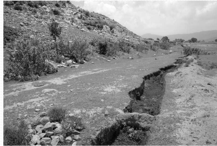
A 'water absorption trench' at the base of a hill in Koilu watershed
